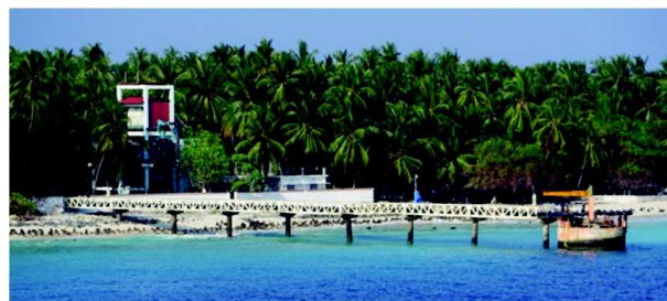
Fig. 2: Low-Temperature Thermal Desalination (LTTD) plant at Kavaratti Island
