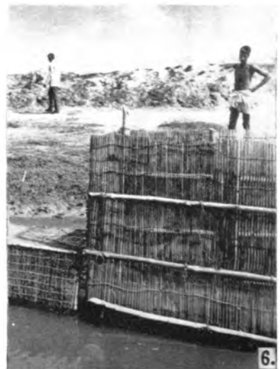
FIG. 1. A general view of a portion of the bheri. .. 2. The feeder canal through which tide water flows into the ponds. .. 3. The sluice box through which water is let in. .. 4. A sluice gate for controlling water supply. .. 5. Bamboo gratings arranged in the form of a 'W' in front of the sluice gate. .. 6. An 'Atol' fixed in the gap between two bamboo gratings, erected in the form of a V.
