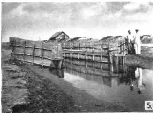
FIG. 1. A general view of a portion of the bheri. .. 2. The feeder canal through which tide water flows into the ponds. .. 3. The sluice box through which water is let in. .. 4. A sluice gate for controlling water supply. .. 5. Bamboo gratings arranged in the form of a 'W' in front of the sluice gate. .. 6. An 'Atol' fixed in the gap between two bamboo gratings, erected in the form of a V.
