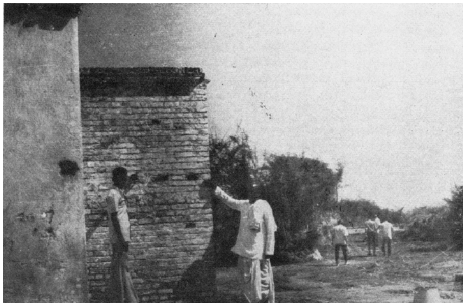
FIG. 3. The priest showing the surge-height against the temple-wall at Hamsaladevi.
