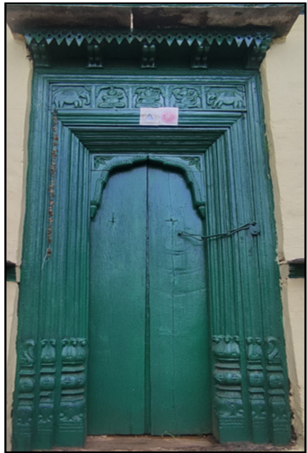
Fig. 4 A Sankal in the main door of the house. ICHR Project work
