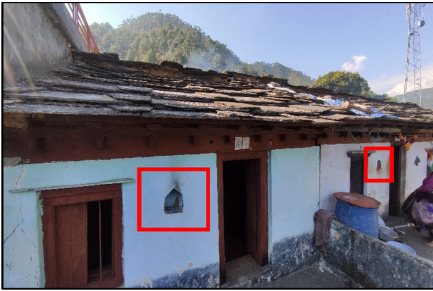
Fig. 9 Jaal/Jav can be seen in the red boxes. ICHR Project work
