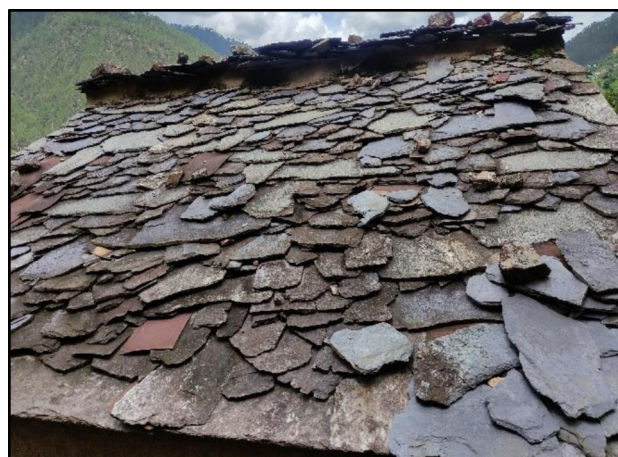
Fig. 2 Patal used on the roof. ICHR Project work
