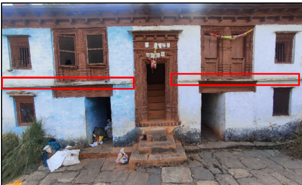
Fig. 10 Sapyal/ Sapeli can be seen in the red boxes. ICHR Project work
