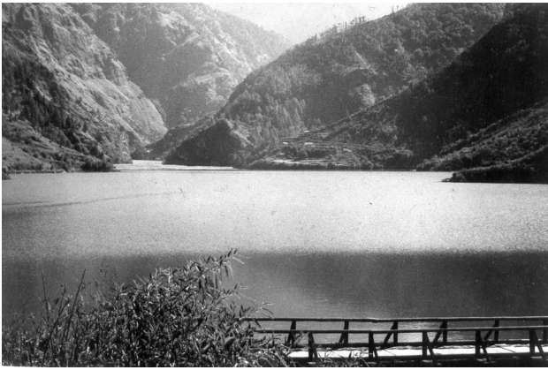
Fig. 5 A view of Gohna Lake from the entrance. A wooden bridge had existed over the outlet of the lake's water, allowing access to Durmi village and the Forest Rest House. (Photo: Author, 1968)
