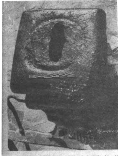
Fig. 10. Top view of the ornamented iron pillar of Delhi showing the fitting of the square iron ring on circular end of the pillar.
