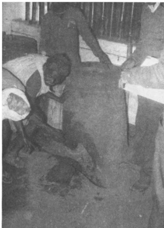
Fig. 5. Bishunpur iron making furnace operated in 1989-90. 17
