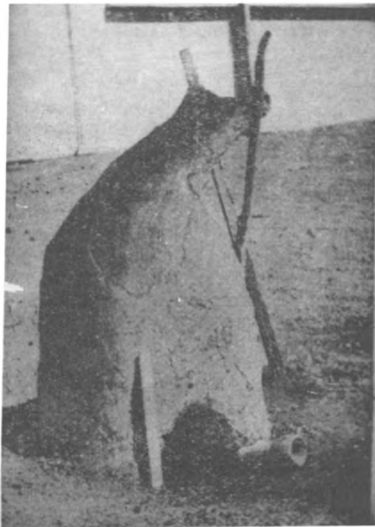
Fig. 4. Jiragora ironmaking furnace operated in 1963. 13
