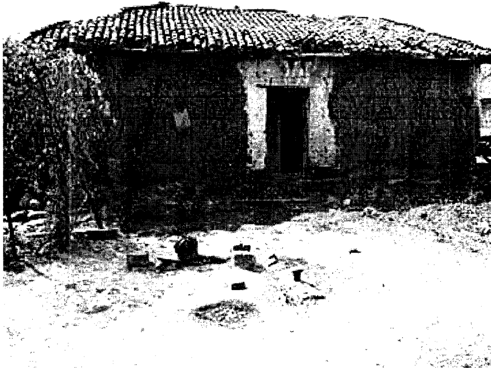
Fig. 1. A blacksmith's house made of slag "bricks" located at Ramgapet in Jagtial mandal, Karimnagar district.
