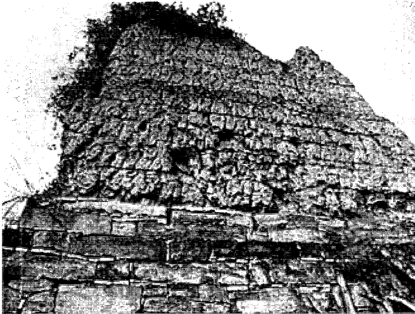
Fig. 3. Slag pieces in mud walls of fortalice.
